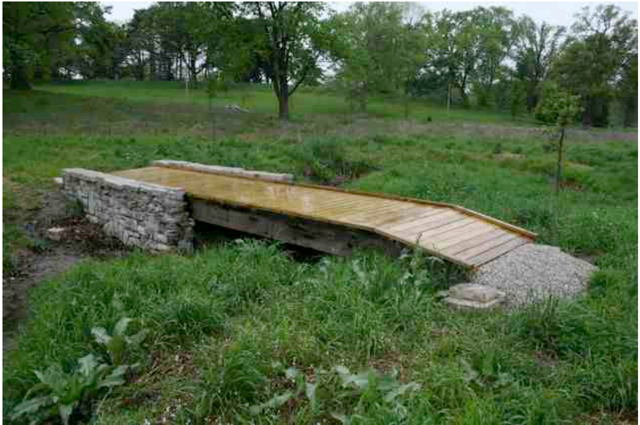
The stone bridge over the creek taken on a rainy day last April
