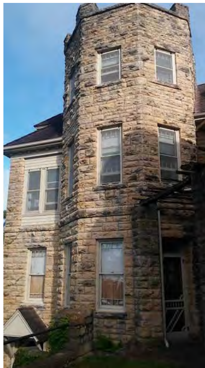
John Bothwell built the tower over a cave to cool the lodge
