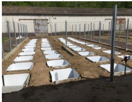
Placing the liners
