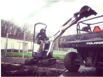
Digging the last of 88 holes!
